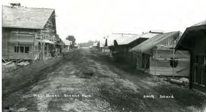
Main Street, Greene Park under construction. (WA State Historical Society )
